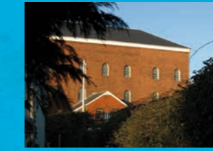
The Pumping Station
