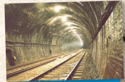
76,400,000 bricks were used to build the tunnel. 28,000,000 came from the two Sudbrook brickworks.
