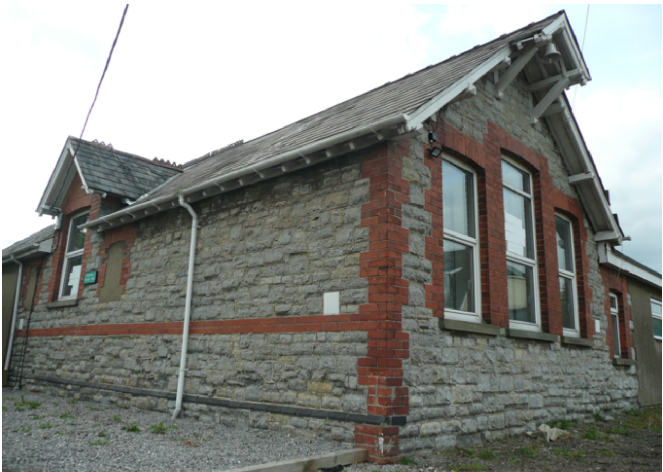
The former Bishton School (Martin Gerrard)
