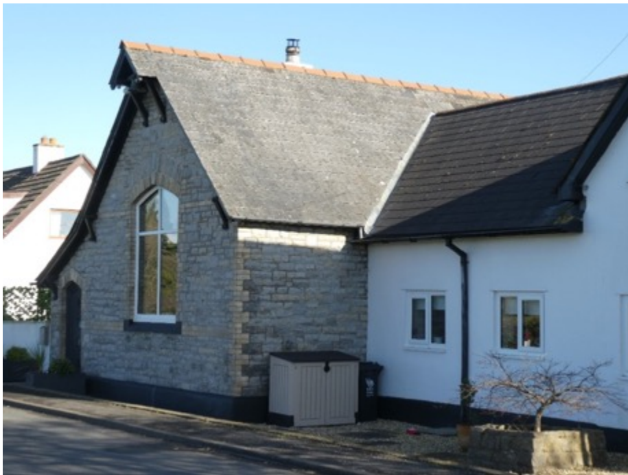
Former school building
