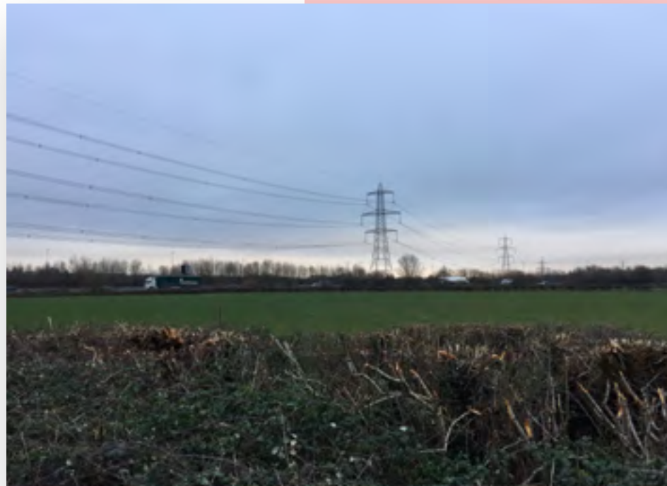
Pylons and motorway into Newport across the Levels; a sign of infrastructure to accommodate a large town or city. ED DREWITT
