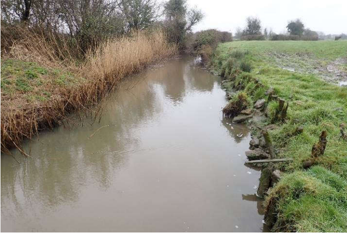
CF1-IDB71 looking SW (19 th March)
