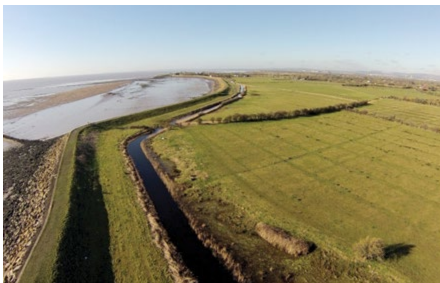
Figure 6. Sea wall re-alignment at Goldcliff. Note how the sea wall has been moved inland leaving a small, triangular remnant of the field in the middle distance.
