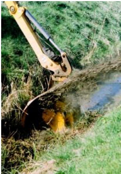
Figure 3: Desilting and spreading using a boom-mounted spreader (Klose Engineering)
