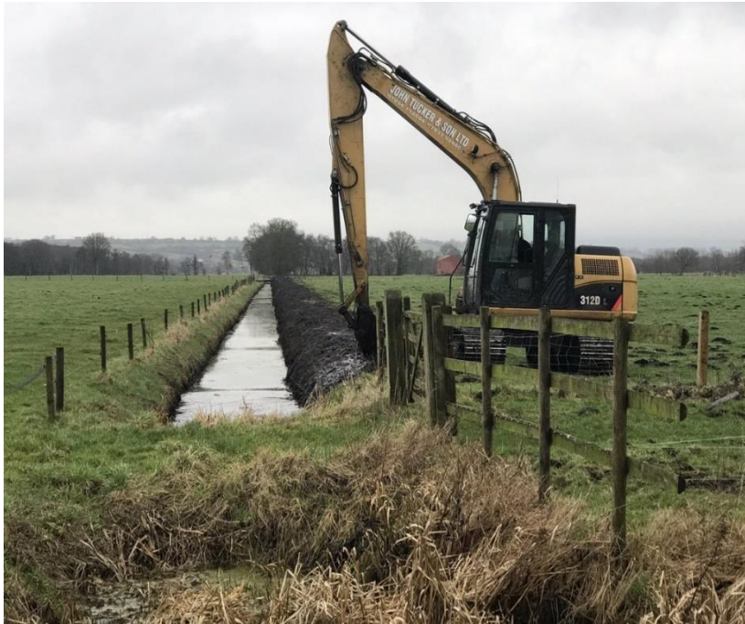
Figure 4: Desilting leaving arisings on bank top
